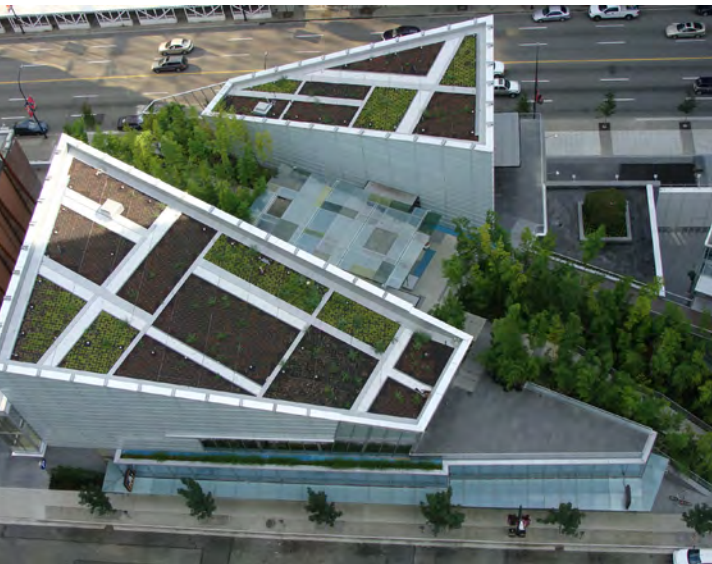
Incorporating green roof technology can reduce the effects of the urban heat island effect and reduce the impact on stormwater infrastructure
