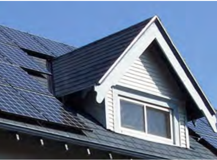
Buildings should be designed to ensure renewable technologies can be incorporated at a later date
