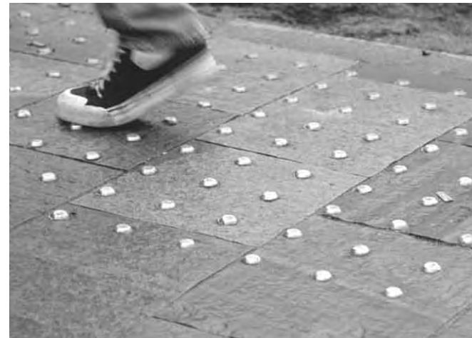
Tactile paving warns the visually impaired of crossings
