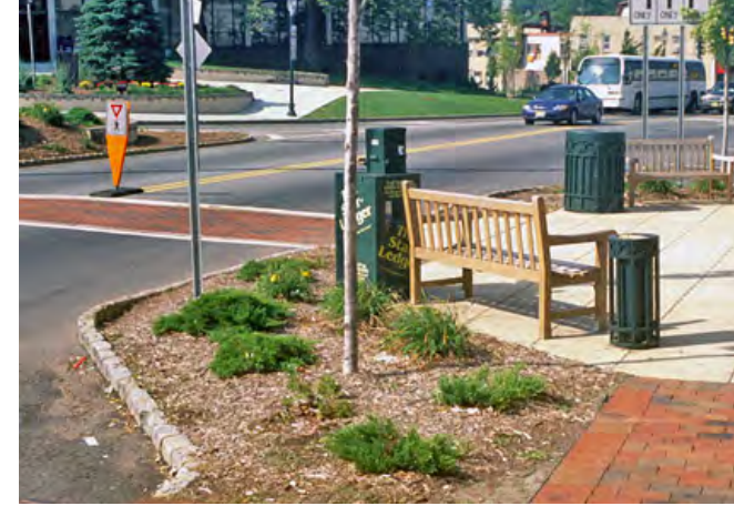
Bulb-outs at key intersections provide a safer crossing for pedestrians
