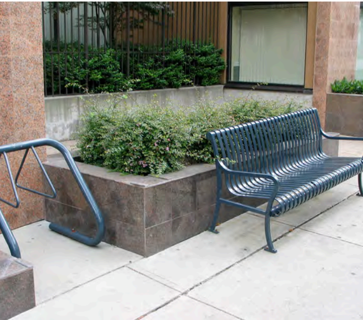
Bicycle facilities should be integrated into the streetscape while allowing for barrier free movement along the street
